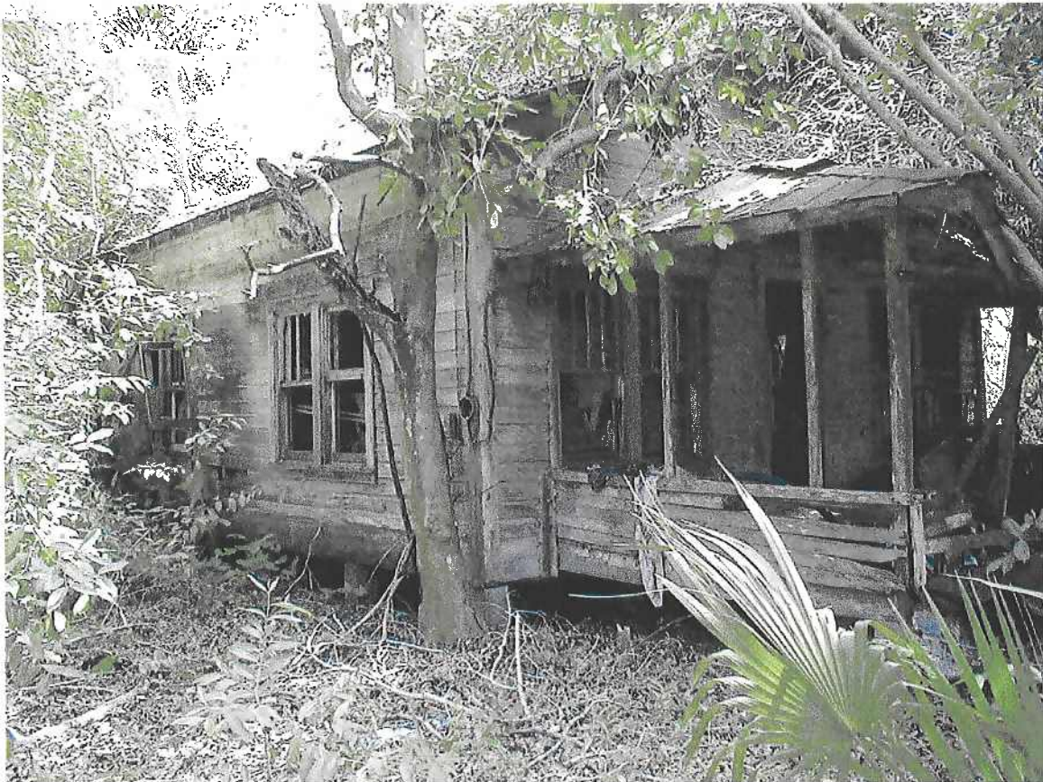
PHOTO 1- ORIGINAL RESIDENCE IN CENTRAL PORTION OF THE SITE
