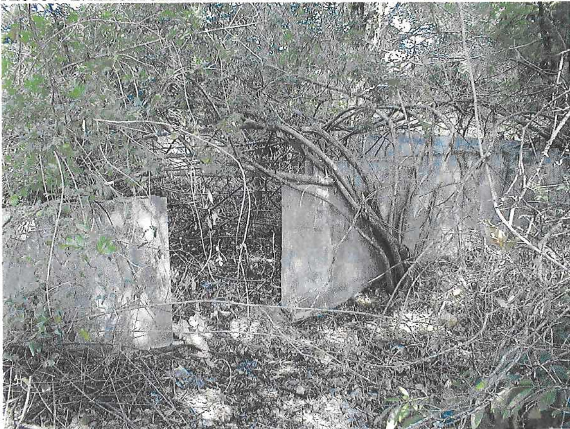
PHOTO 6 - UNFINISHED CONSTRUCTION PROJECT
