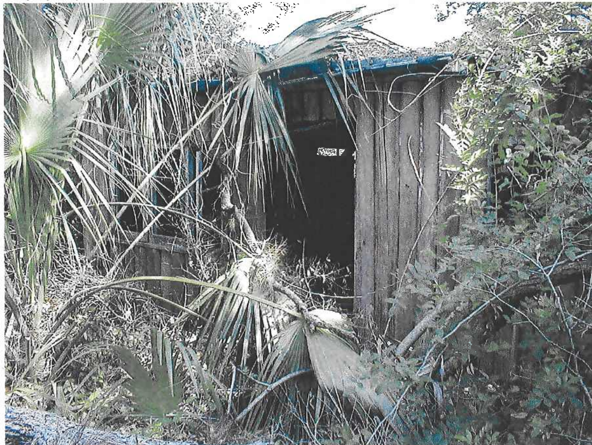
PHOTO 2 - LOG HOME NORTH OF THE MOBILE HOME
